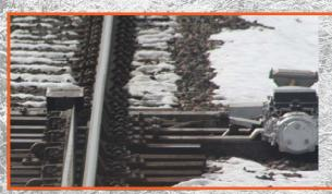
Nearly **5,000** switch heaters are in place to ensure remote-controlled rail switches do not freeze.
